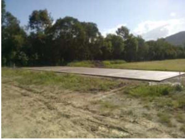
Slab down - we're on the way
