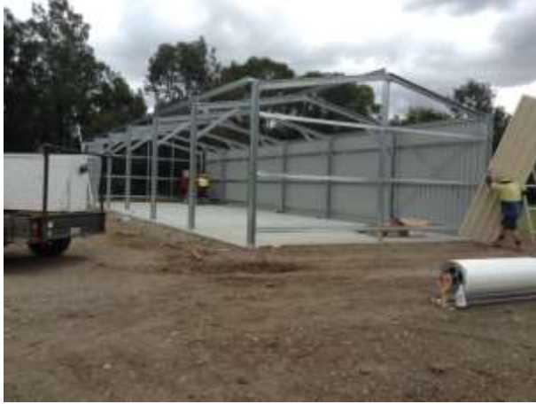
Erection well on the way
