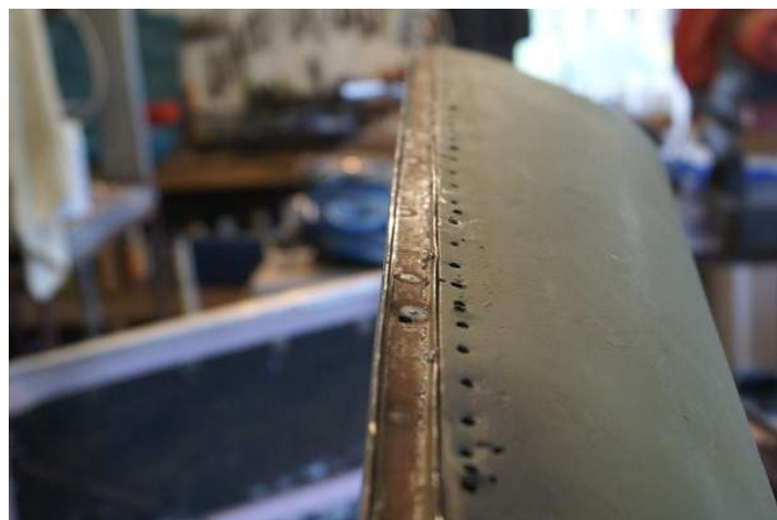
Water exclusion channel in situ
