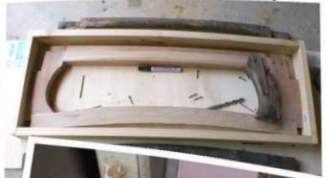
Rear window timber in framing box
