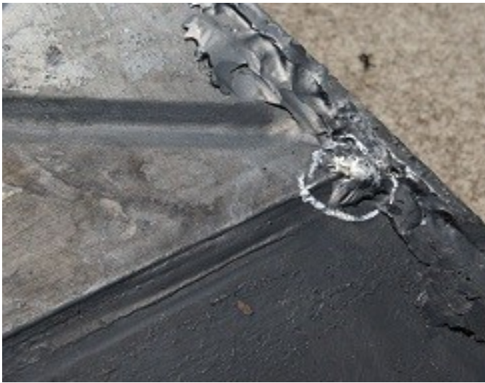
Above: Resoldered seam
